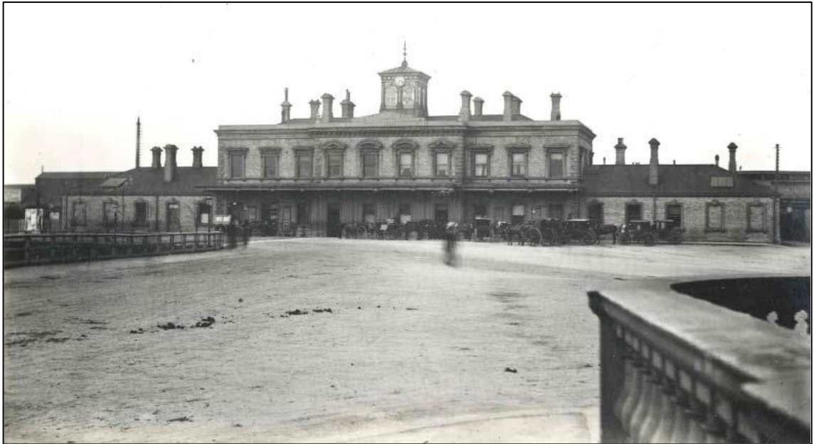
Fig 23: Reading General Station c. 1900
